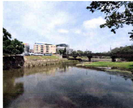
Fig. 10 - View of the site and Bernie Banton Bridge, looking upstream from north bank. Source: JPW Site Photo
